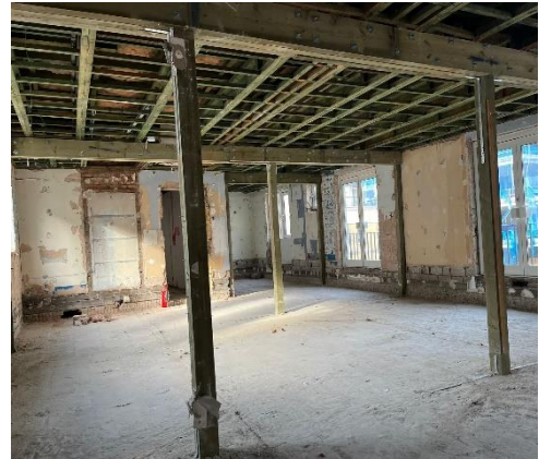
Internal stripped out areas
