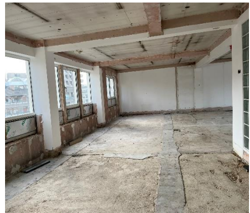
Internal stripped out areas
